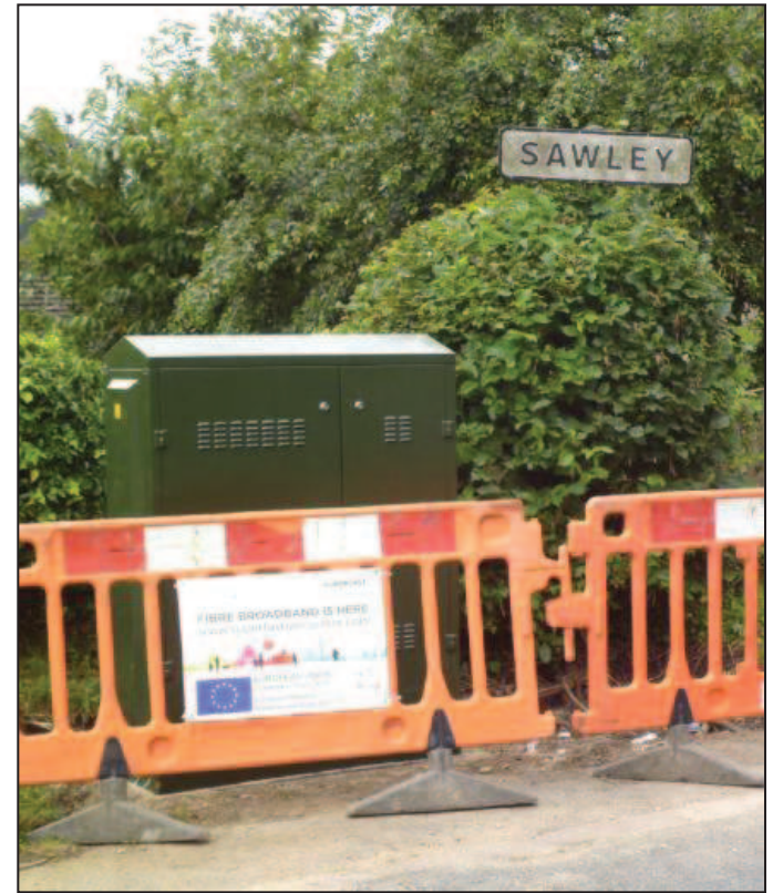
Cabinets in the villages of Chatburn and Sawley, in the process of build.
