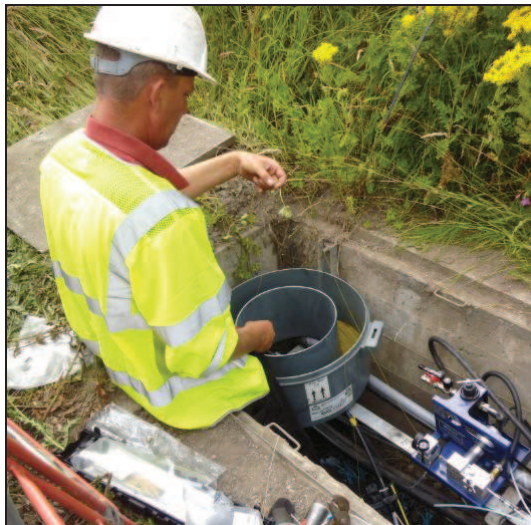
Fibre distribution network splicing in Blackburn
